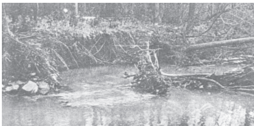
Fig. 17.6: Stream bank erosion
