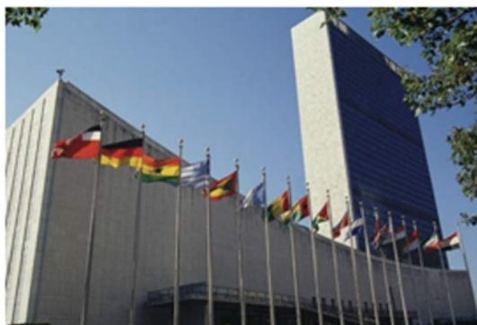
Figure 27.4 UN Building, New York
