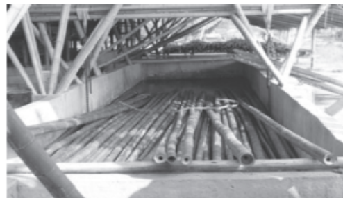
Fig. 6.8: Soaking bamboo in a water tank
