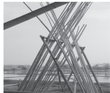
Fig. 6.6: Standing the bamboo poles
