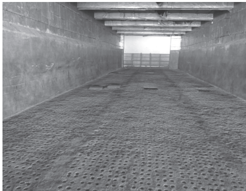
Fig. 11.6: Side cross section of tunnel with plenum
