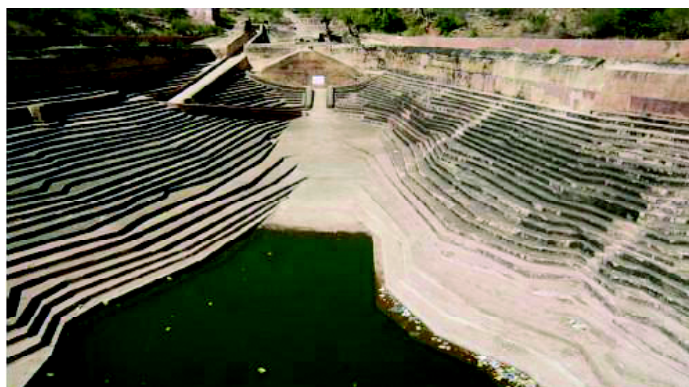
Fig. 16.6 : A Traditional Method of Rainwater Harvesting
