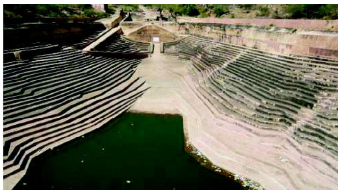
Fig. 16.6 : A Traditional Method of Rainwater Harvesting
