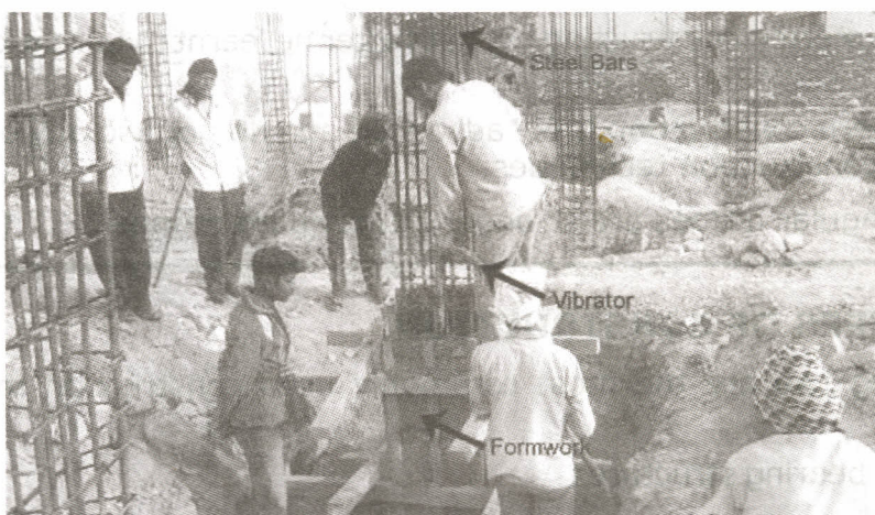
Fig: 6.3 Image showing laying process of cement concrete with steel bars in rcc column
