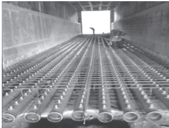
Fig. 3.9: Tunnel with pipes and spigots (under construction)
