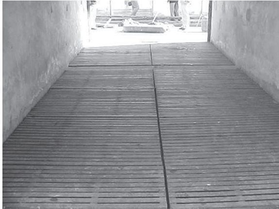
Fig. 3.8: Tunnel with iron grating
